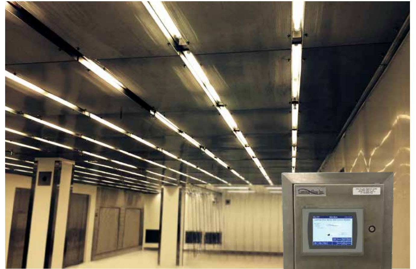
HMI TOUCHSCREEN INTERFACE PLC
